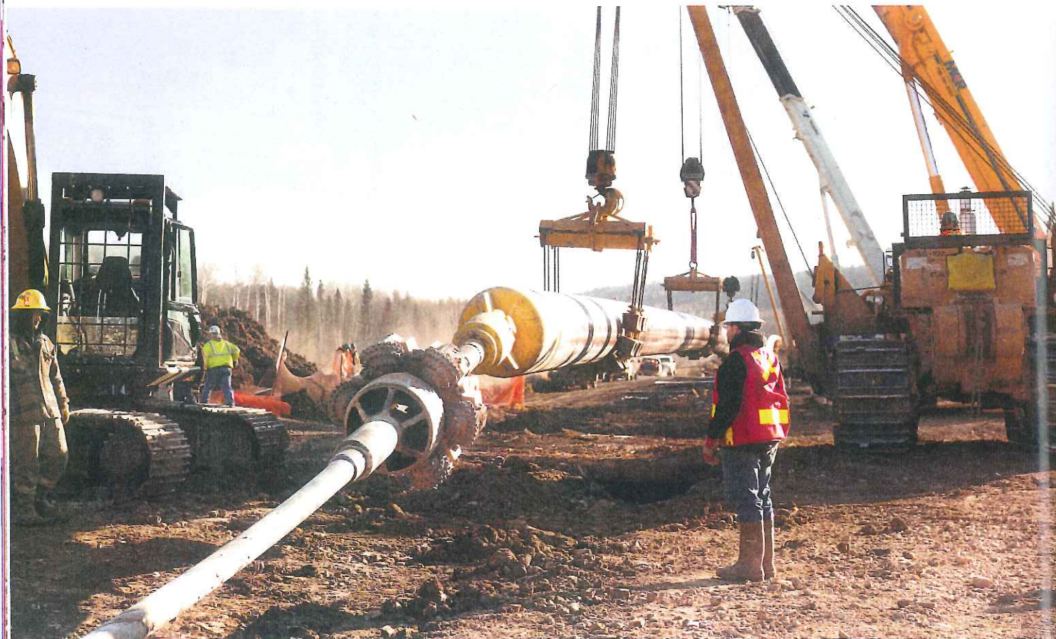
After a tunnel was drilled under the Clearwater River, a swivel is attached to the pre-assembled pipe section. The swivel will pull the pipe through the drilled underground tunnel.
