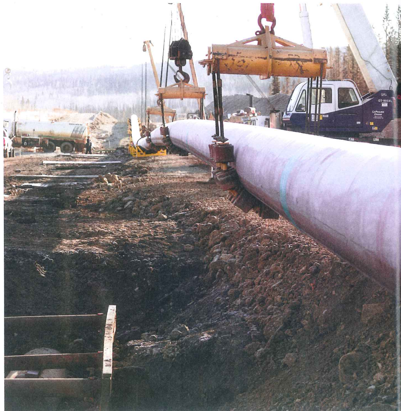
Cranes use roller cradles to support a welded section of pipe during the Clearwater River horizontal directional drill pull back operation.
